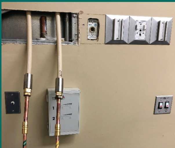
Flameless addition of medical gas outlets
